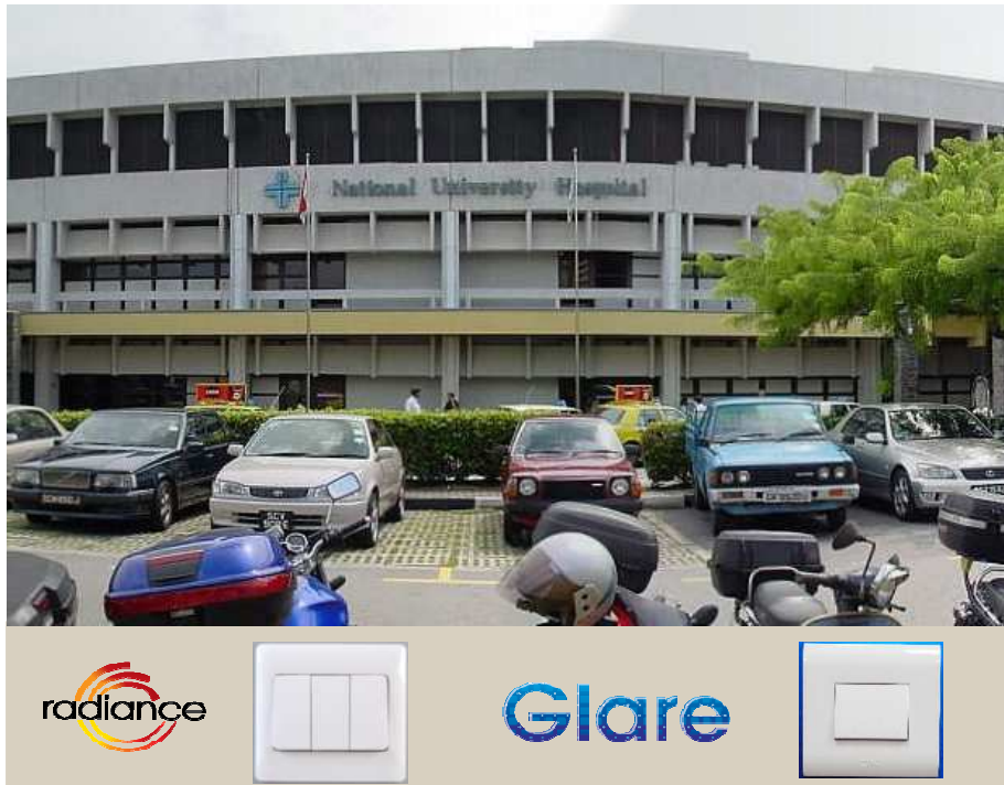
NUH - Remodeling of wards and refurbishment to ICUs
